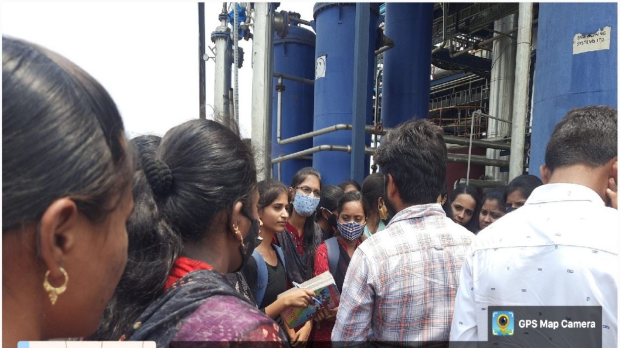
Oxygen plant Head Mr. Sanjay Patil explain working of plant
